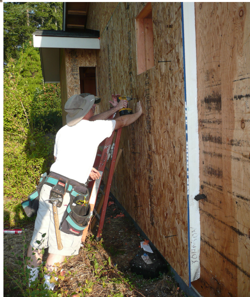
(Left) Installation crews created an airtight envelope using expanding foam between panels and around window openings. (Below) Specialty SIP screws were used to attach retrofit insulated panels to the existing studs.
