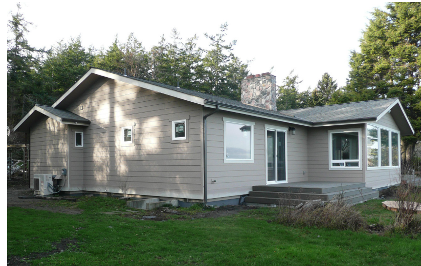
Installing retrofit insulated panels, roof insulation and new windows helped cut the home’s heating cost by 83.5 percent
