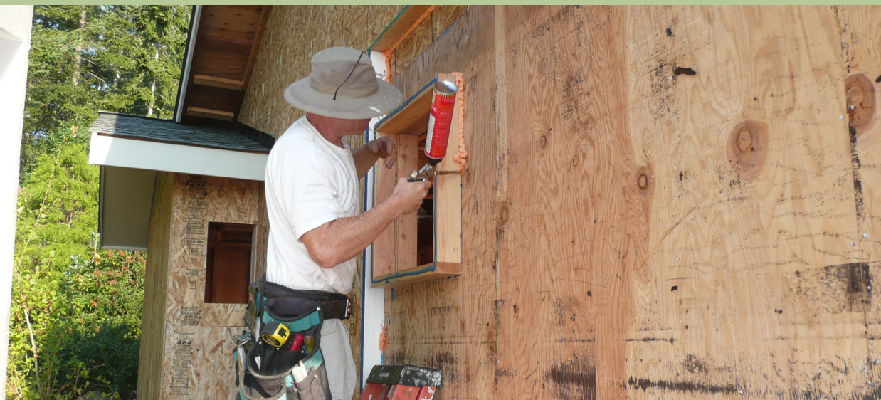
(Left) Installation crews created an airtight envelope using expanding foam between panels and around window openings. (Below) Specialty SIP screws were used to attach retrofit insulated panels to the existing studs.
