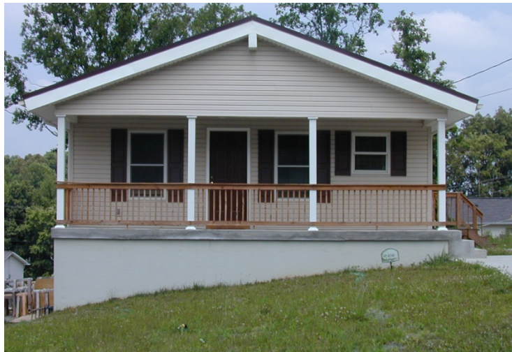
Fig. 3. East elevation of ZEH5 from the street.
