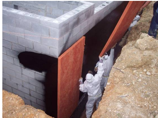
Fig. 23. Installation of 4 × 8 ft fiberglass boards sized to cover the waterproofing.
