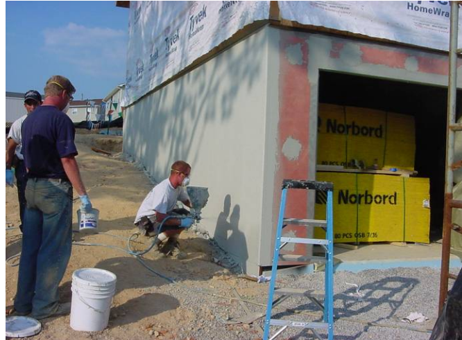
Fig. 25. The above-grade portion of the foundation wall receiving final spray covering.
