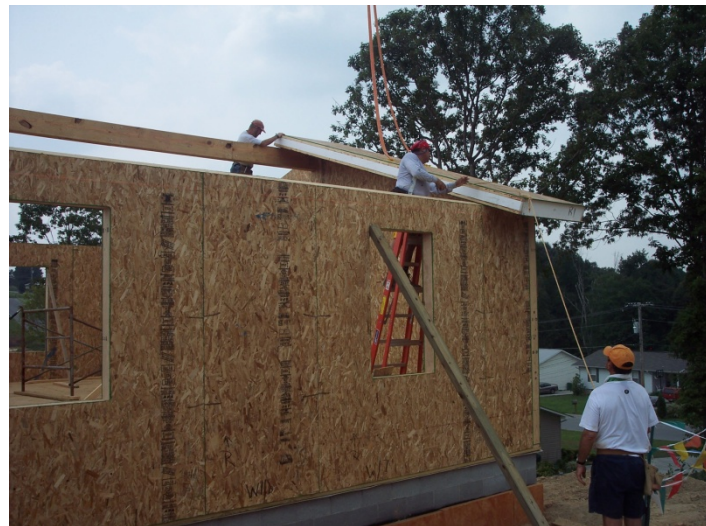
Fig. 33. The SIP roof panel installation.
