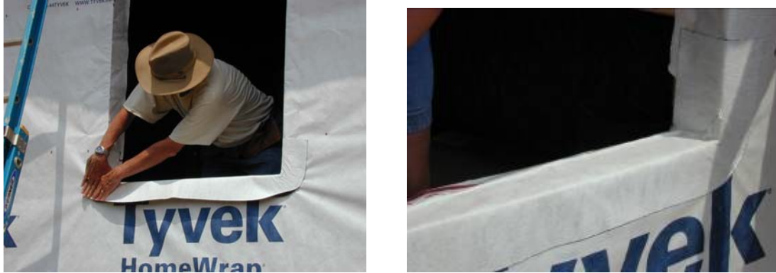
Fig. 29. Panned window opening.
