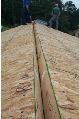
Fig. 41. Space above the ridge beam is used for a wiring chase.
