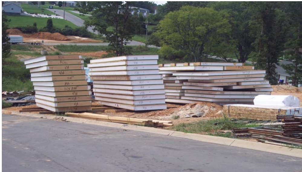
Fig. 4. Structural insulated panels (SIPs) for ZEH5 come numbered to match the panel cut drawings. SIP should be stacked in the order in which they will be installed.
