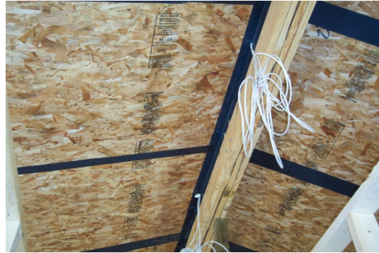
Fig. 42. Wires being pulled into the space above the ridge beam.
