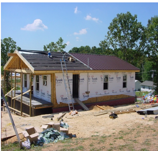
Fig. 30. Roof drainage plane under the raised metal roof. (See Appendix B, Resources.)
