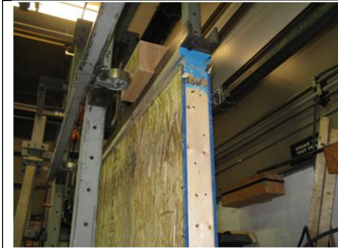
Figure E5. Typical failure mode of walls with a combination of nail head pullout, pull-through and nail withdrawal from wall perimeter, as well as top plate coming unattached to wall studs (Figure E4).
