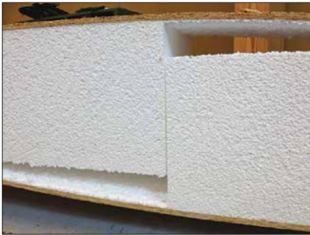
Figure 12. Adhesion failure (FPL).
