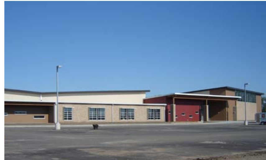
SIPs and other energy-efficient features are estimated to save the school district 30 percent in utility costs.
