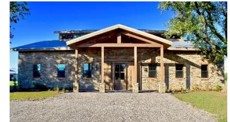
Describe the benefits of using SIPs on this project. Did SIPs help save time, labor, construction costs, or energy? SIPs provided energy efficiency, sound control, a shorter construction time, overall interior comfort, ability to regulate interior thermals (especially for the MRI area), and improved performance of HVAC system. The SIP construction provided a very energy efficient envelope that was very stable, so the only design challenges were driven by the fluctuating internal loads.
