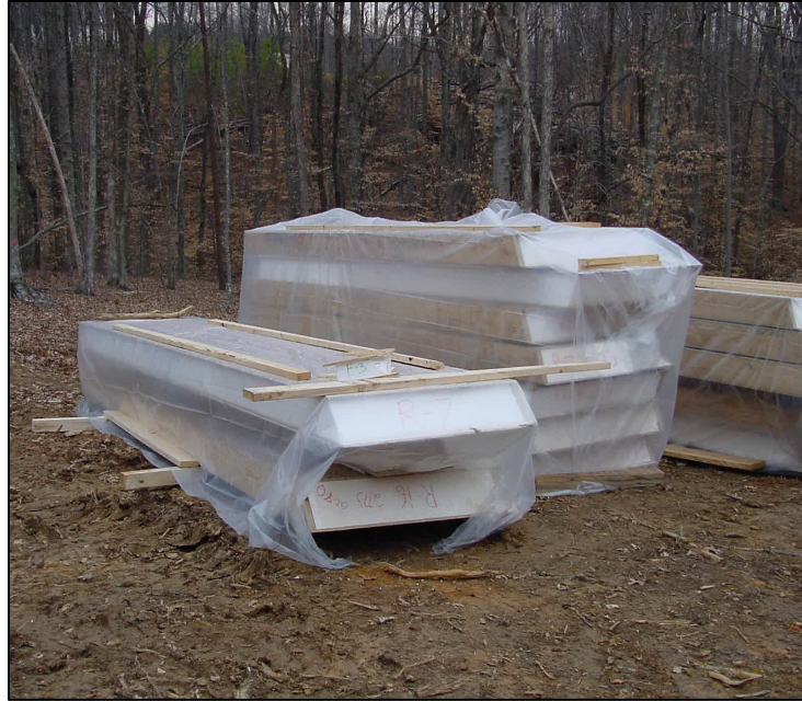
Figure 2: SIPs stored off the ground, level, and protected from the elements
