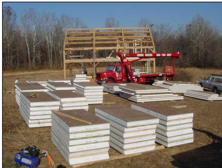
Figure 1: Staging area for panel sorting and prep
