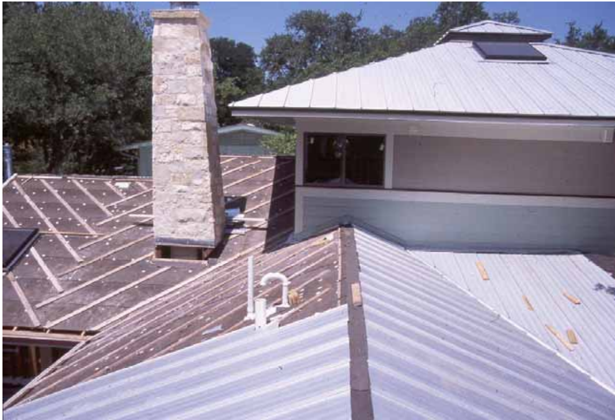
Diagonal lath under metal roofing
