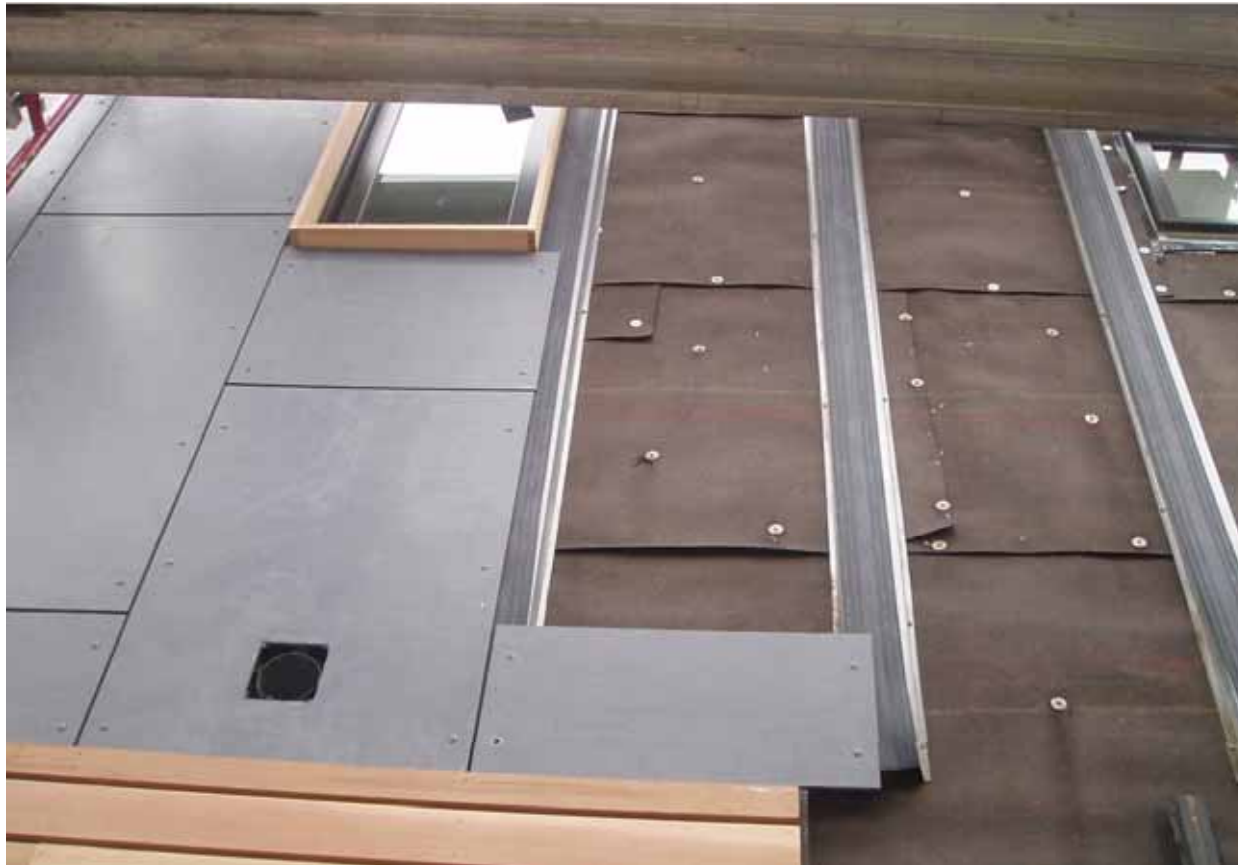
Drainage plane with ventilated cladding
