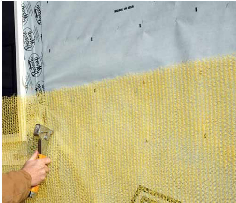
Ventilated cladding with drainage mat
