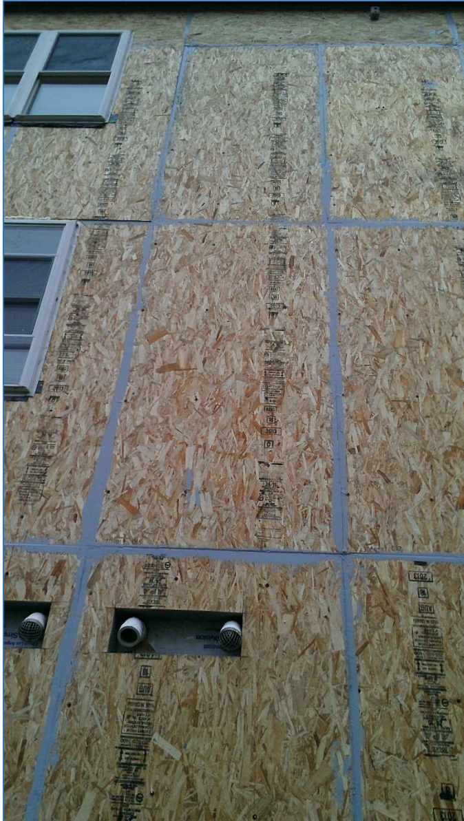
Figure 20. Large Rectangular Cutouts to Accommodate Water Heater Direct Vent Piping
