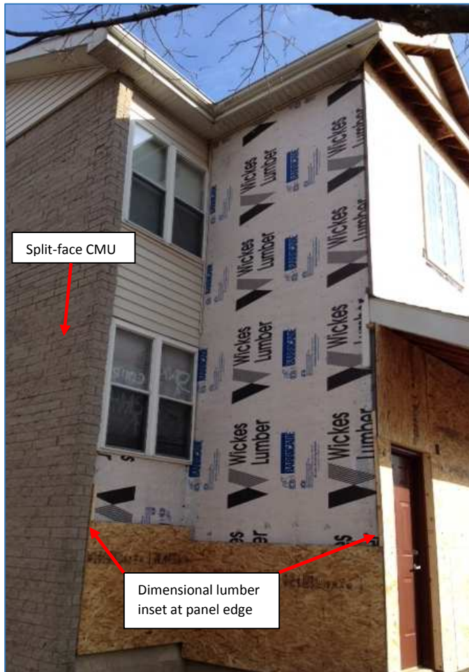
Figure 8. West Northwest Exposure, Left Side Elevation
