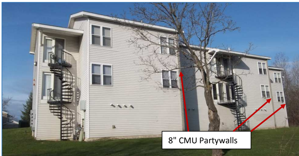
Figure 4. Rear Elevation (northeast), 150 Lark
