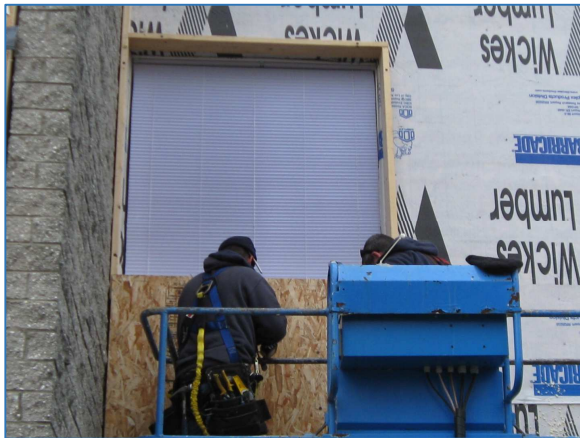
Figure 11. Window Jamb Extensions Were Formed with 2x6s Applied from the Exterior
