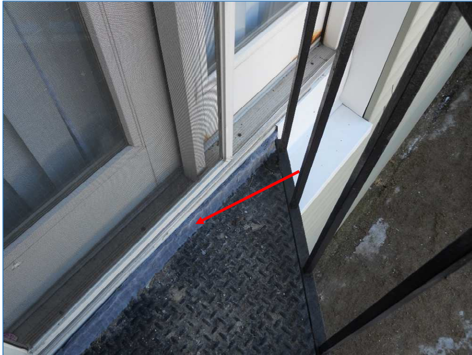
Figure 18. Aerogel Fabric between Stair Landing and Band Board below Door
