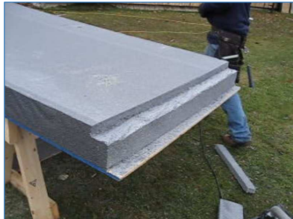
Figure 15. Panel Edge Grooves for Inverted Ledger
