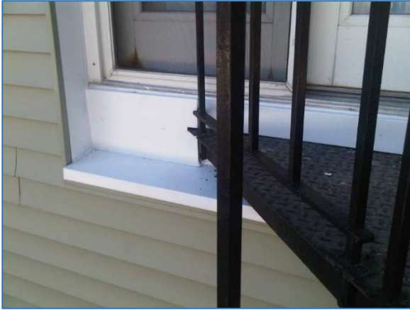
Figure 16. Patio Door Band Board behind Stair Landing Completed
