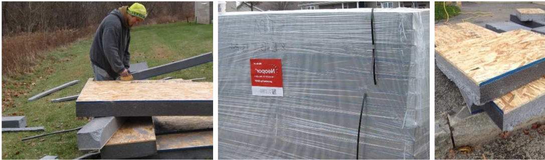
Figure 1. Six-inch Retrofit Insulating Panels
