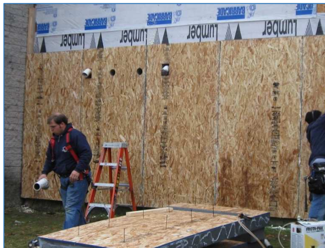
Figure 19. Application of Panel-to-Panel Adhesive
