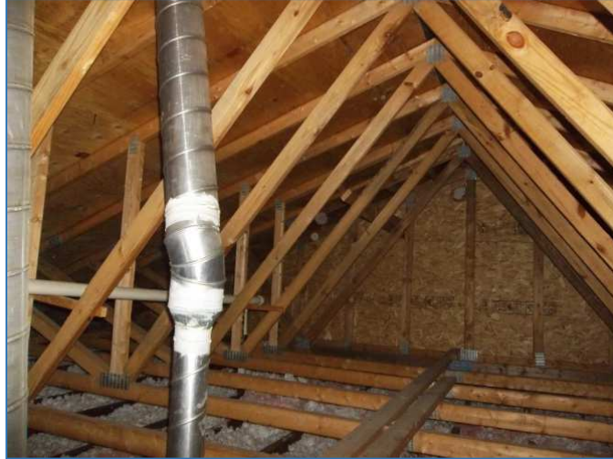
Figure 5. Typical Attic at East End of Building
