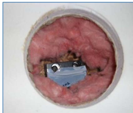
Figure 7. Sensor Fastened within Existing Wall Cavity Via Hole Cored in Drywall
