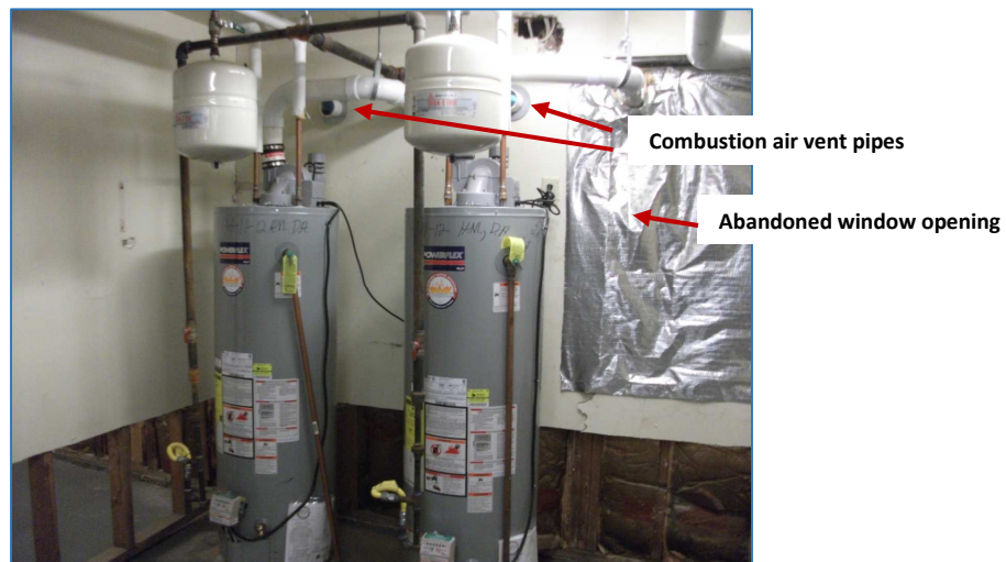
Figure 6. Typical Water Heater Installation for Two or Three Apartments
