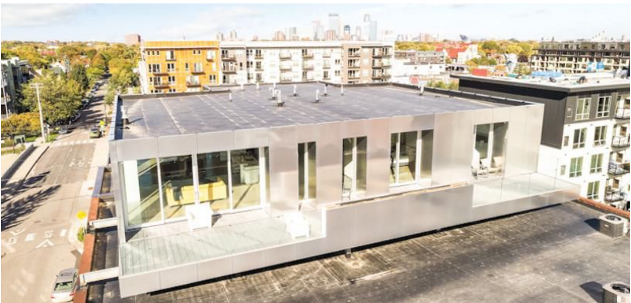
The Bryant Residential Loft scored 0.80 ACH50 on the blower door test, significantly lower than the Climate Zone requirement and key to keeping outdoor pollutants diluted. Credit: Courtesy of Energy Panel Structures
