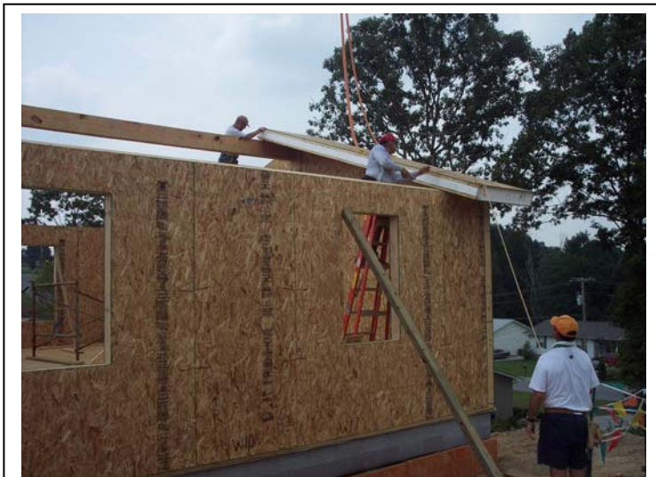
Figure 32. The SIP roof panel installation.
