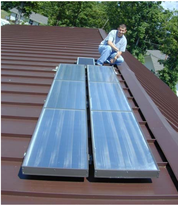
Figure 49. SolarRoofs, SkyLine System 5 solar water heater, with 38 ft 2 of solar collector area installed on the roof of ZEH5.
