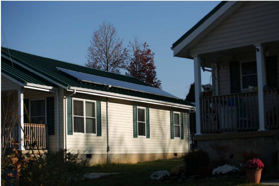
Figure 45. Solar modules sit nicely on the roof of ZEH2. The dark green roof makes for a very pleasing appearance with the dark bluish-green polycrystalline module.
