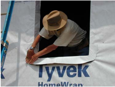
Figure 28. Panned window opening.
