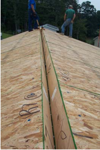
Figure 39. Space above the ridge beam is used for a wiring chase.
