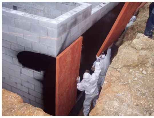
Figure 22. Installation of 4 x 8-ft fiberglass boards sized to cover the waterproofing.
