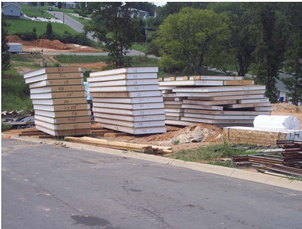
Figure 5. SIP panels for ZEH5 come numbered to match the panel cut drawings. SIPs should be stacked in the order in which they will be installed.
